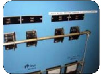
Photo 2 : Lock Out/Tag Out notice on ship equipment panel.
